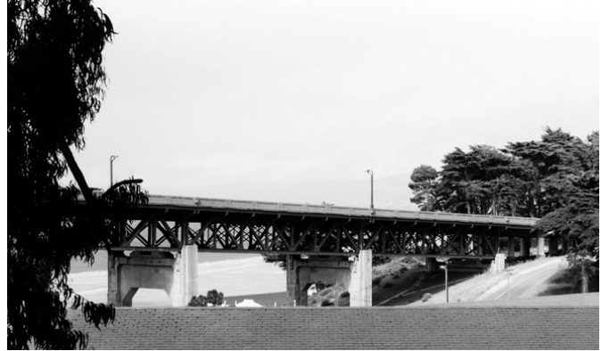
Doyle Drive viaduct structure
